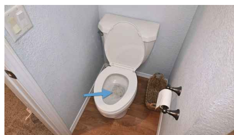
Basement Bathroom Clogged By Toilet Paper
