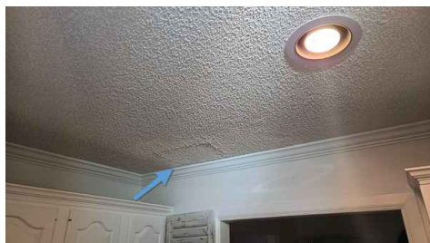
1st Floor Kitchen
