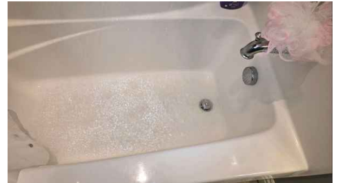
1st Floor Hall Bathroom Tub
