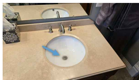
1st Floor Hall Bathroom Right Sink
