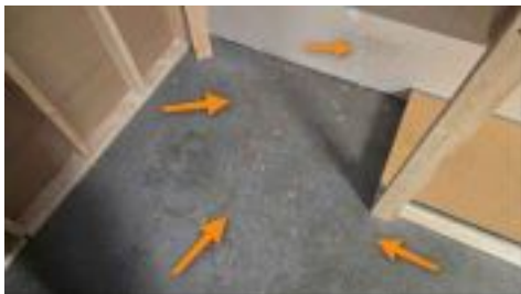
In Basement Below Master Shower
