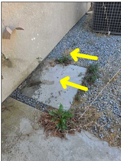
Potential for ponding water
