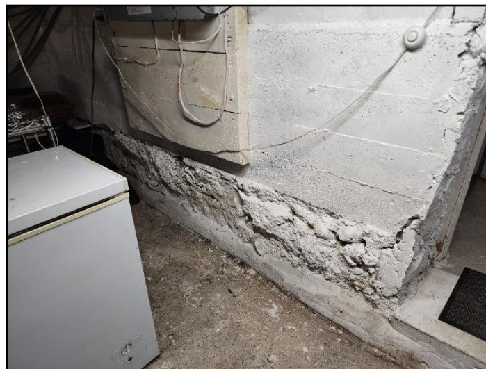
10. Basement lowered or underpinned
