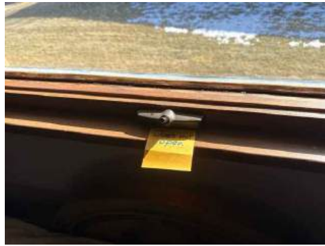
1st Floor Bedroom Window Unable To Test Close Up
