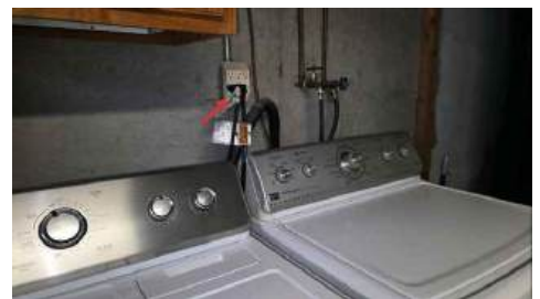
Basement Laundry Room
