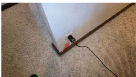
1st Floor Dining Room Outlet
