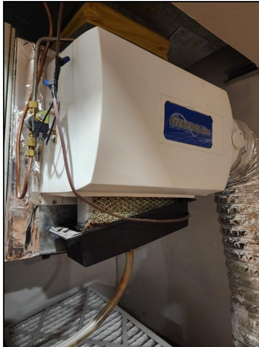
21. Clean pad/mesh - regular maintenance
