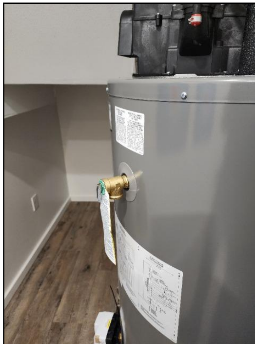
32. Discharge tube missing
