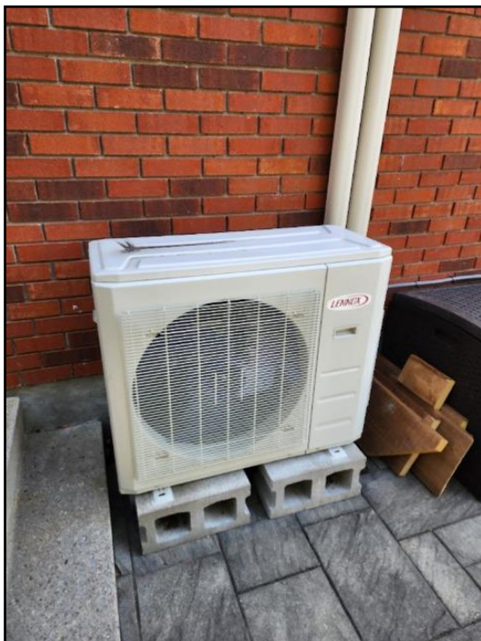
23. Ductless (Mini split) system
