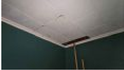
1st Floor Kitchen
