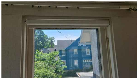
2nd Floor Sun Room
