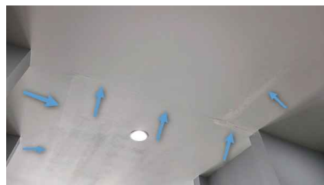
1st Floor Hall
