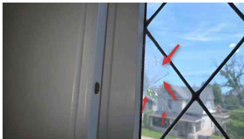
1st Floor Hall
