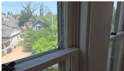
2nd Floor Sun Room
