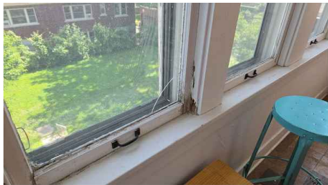
2nd Floor Sun Room
