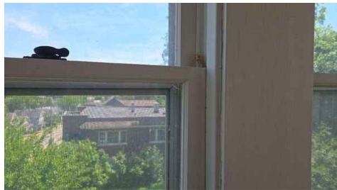
2nd Floor Sun Room
