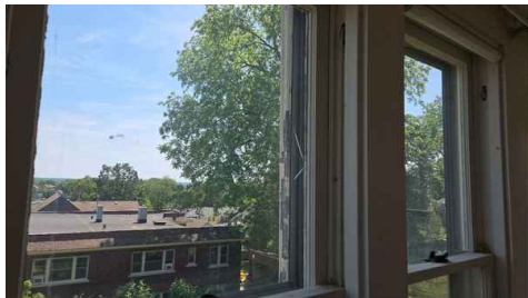
2nd Floor Sun Room
