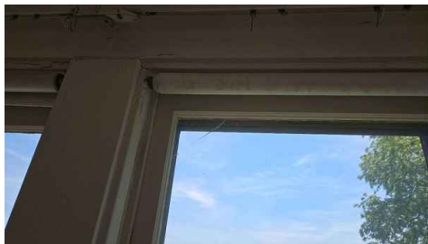
2nd Floor Sun Room
