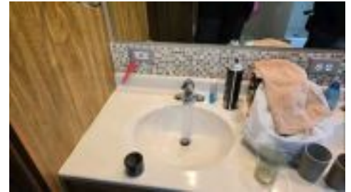
1st Floor Master Bathroom Outlet
