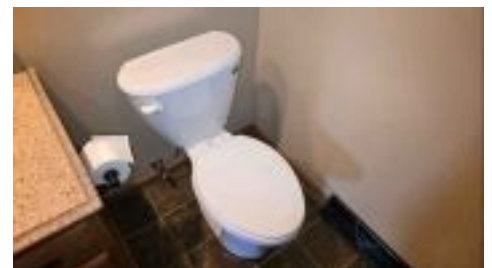
1st Floor Hall Bathroom Toilet
