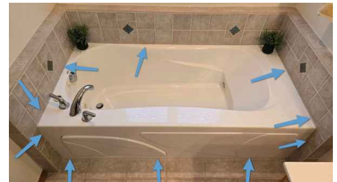
1st Floor Master Bathroom Tub Deteriorated Grout
