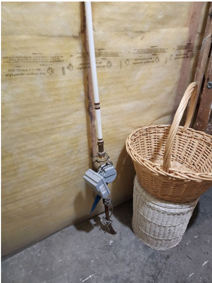
Main water shut off
