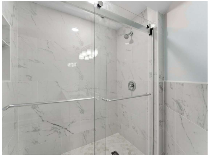
Koehler shower doors. Schluter flooring system in shower to prevent leaking
