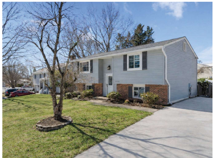
Recent concrete driveway providing access to the studio & backyard. Roof believed to be from 2024
