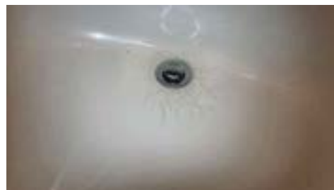
1st Floor Hall Bathroom Sink
