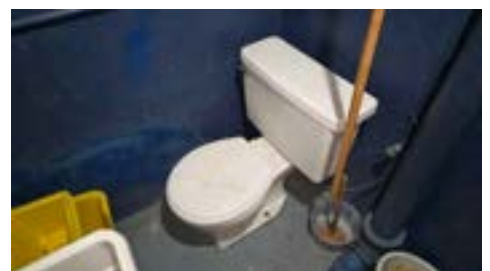
Basement Bathroom Toilet
