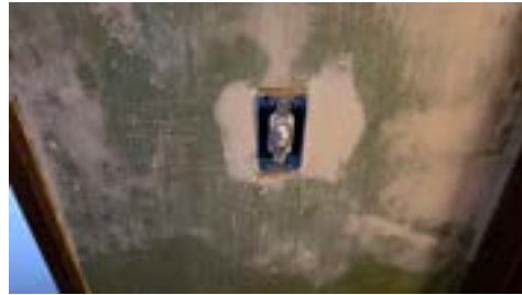
2nd Floor Hall
