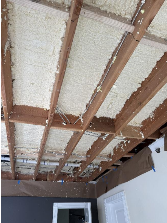
Detailed view of the insulation installed within the original ceiling cavities.
