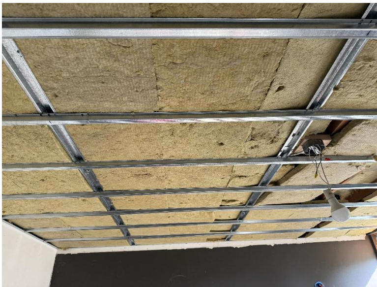
The new ceiling assembly during construction, before installation of the finished drywall surface.
