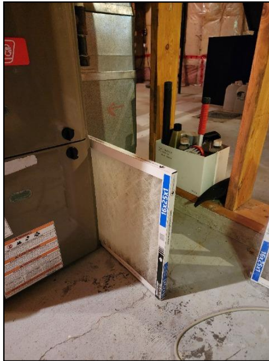
19. Replace - regular maintenance
