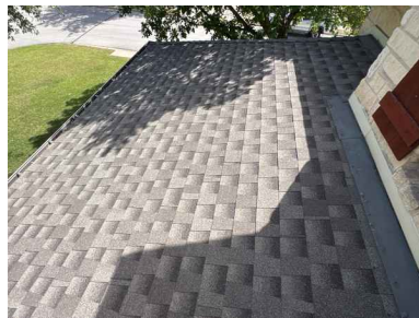
View of the front left corner roof covering above the front porch
