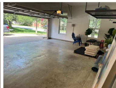
Front right corner measurement not taken due to the slope of the garage
