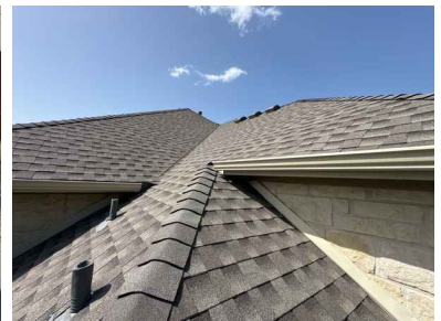
View of the upper front left corner roof covering
