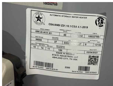
Data plate information for the left side water heater
