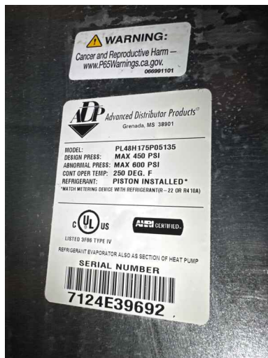
Data plate information for the downstairs air handler
