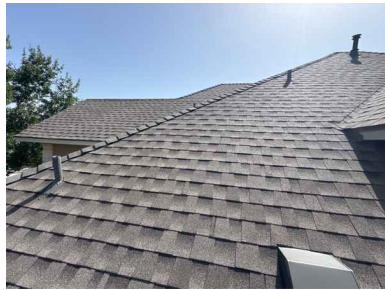
View of the front right side roof covering
