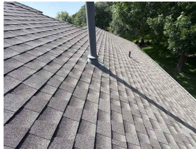
View of the back right side roof covering
