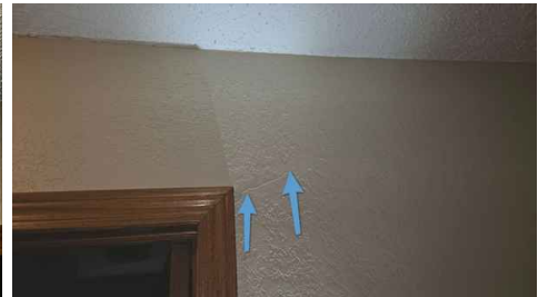
1st Floor Hall On The Top Right Of Bathroom Door
