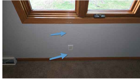
1st Floor Livingroom Under Left Side Of Windows
