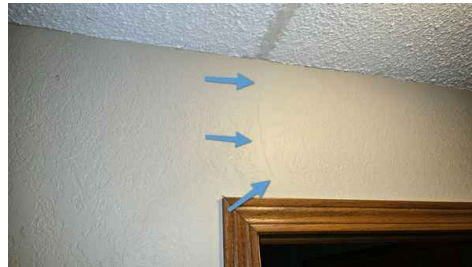
1st Floor Hall Above Bathroom Door
