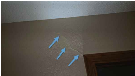
1st Floor Hall Above First Bedroom On The Rights Door
