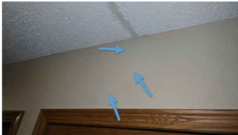
1st Floor Hall Above Closet Door On The Right
