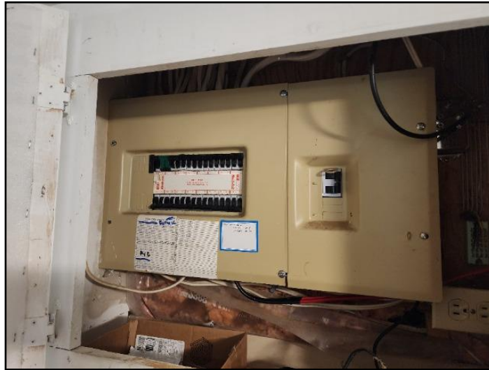
10. Main electrical disconnect
