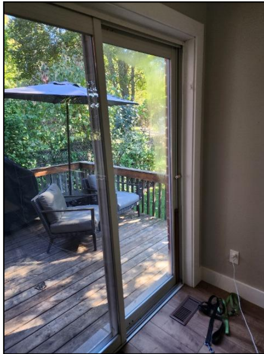
33. Lost seal on double glazing
