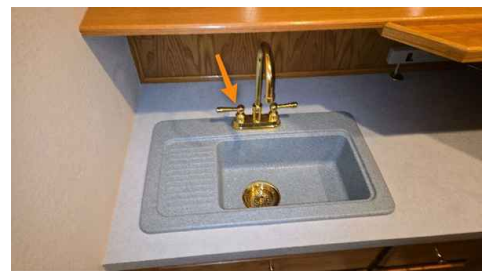
Basement Livingroom Wet Bar
