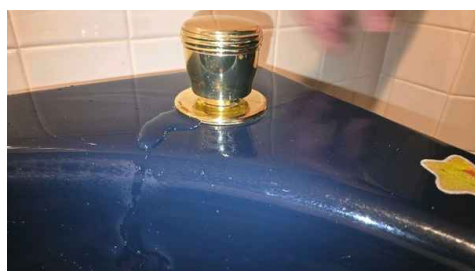
Basement Bathroom Tub Handle Leak
