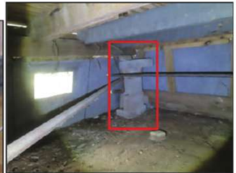
Poorly supported beam(front right corner)
