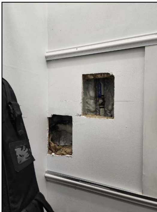
29. Main water shut off
