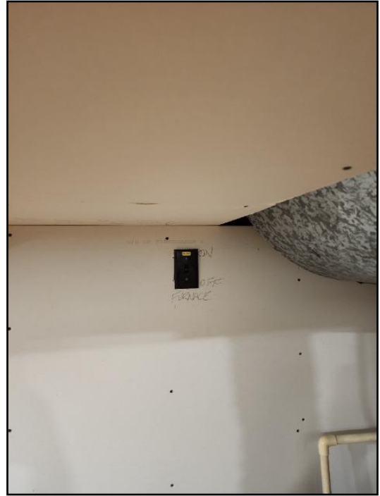
15. Electrical disconnect
