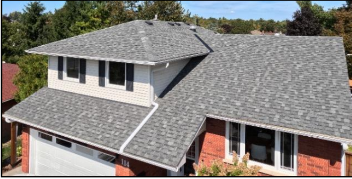
1. Asphalt shingles
