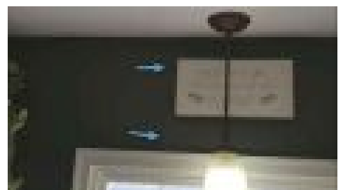
1st Floor Kitchen Above Window
