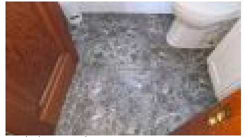
2nd Floor Bathroom
