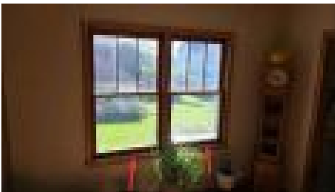
1st Floor Dining Room Windows
