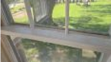
1st Floor Sun Room Windows Missing Locks
