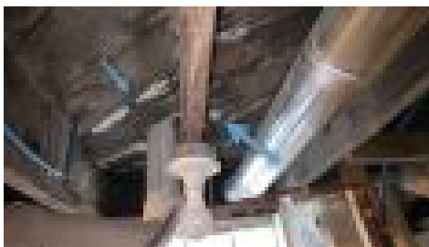
Basement Under 1st Floor Toilet
