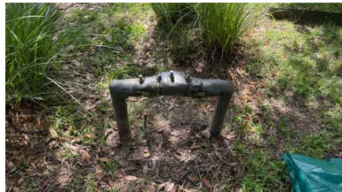
Photo of Irrigation Valve, Backflow Prevention, and Rain Sensor:
