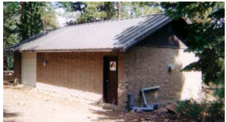
Water Treatment Plant for the Barton Flats Camping Association
