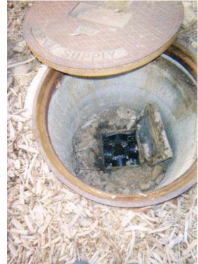
Typical Septic System Distribution Manhole
