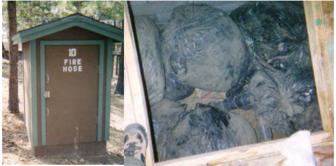
Typical Fire Hose Storage Shed and View of Below Ground Piping With Bags of Insulation
