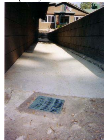
Storm Drain at Wolf Lodge
