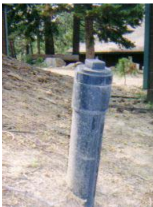
Typical Wastewater Cleanout Riser
