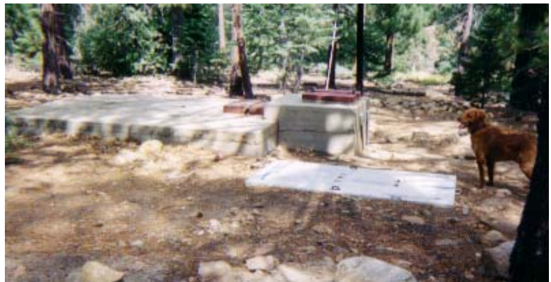
Below Ground Storage Tank at the Water Treatment Plant
