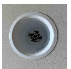
• Outlet cover plate screws appear to be too long. Replace with shorter screws so that the cover plate is properly secured. (**Primary Bathroom**)
